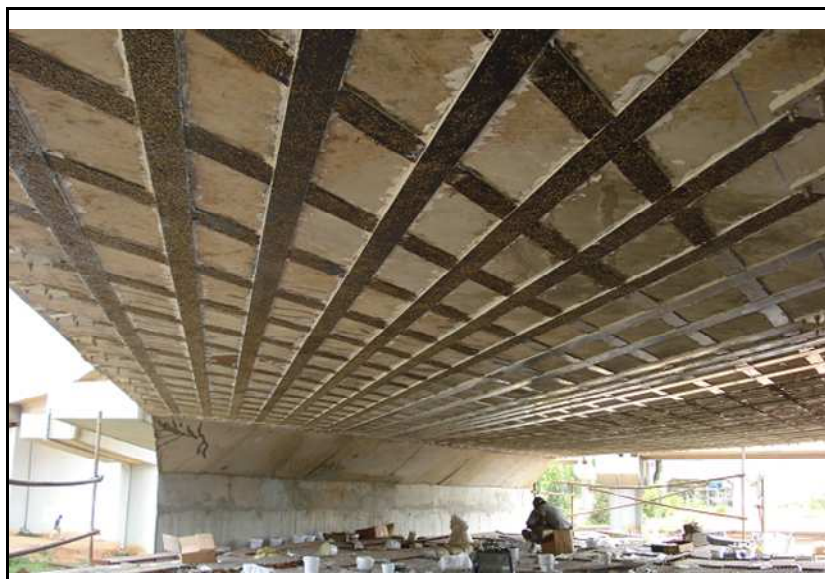
Figure 2: Strengthening of Skew slab using FRP laminates
