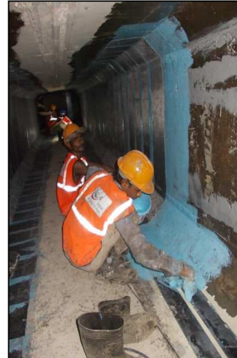
Figure 10: CFRP fiber wrapping being done for shear strengthening of girders
