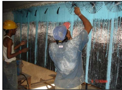
Figure 6: Enclosing the girders with carbon fiber wrapping 5
