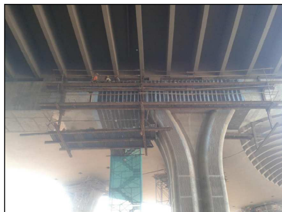
Figure 12: Strengthening of pier caps
