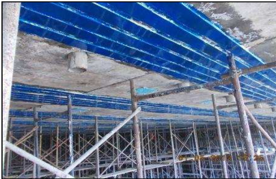
Figure 9: FRP laminates placed for flexural enhancement
