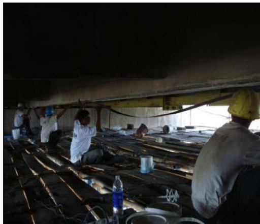
Figure 4: Prestressing in process for the girder 5
