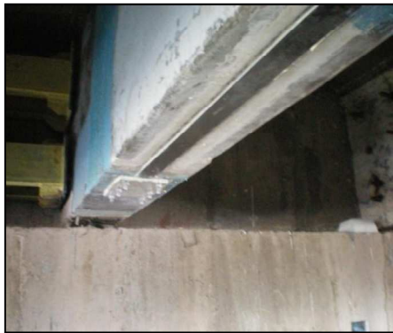
Figure 5: Prestressed laminates with anchor plates at the ends 5
