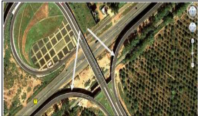
Figure 1: NH7 Highway site
